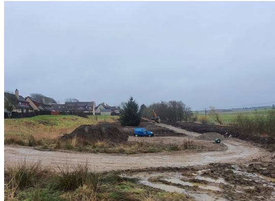
Figure 6 - groundworks commence at the allotment site
